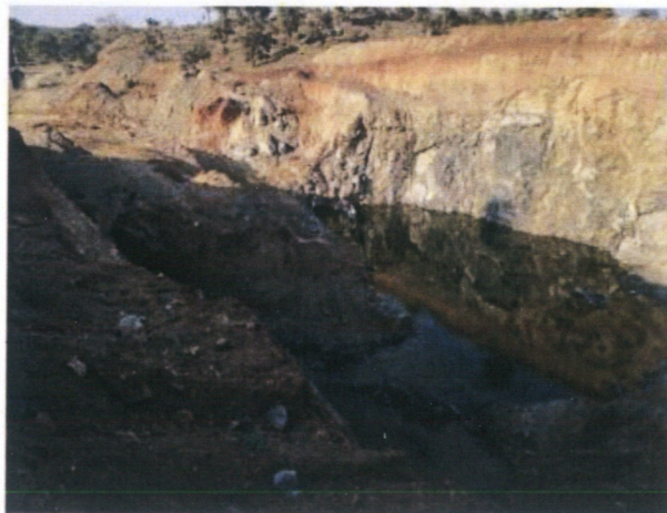
Figure 7:- Water logged pit.
